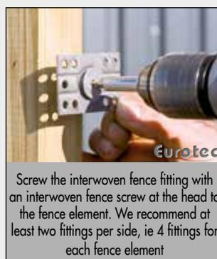
Screw the interwoven fence fitting with an interwoven fence screw at the head to the fence element. We recommend at least two fittings per side, ie 4 fittings for each fence element
