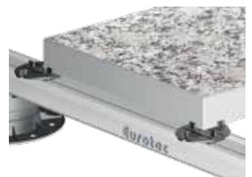
**7** Insert first stone slab and check spacings
