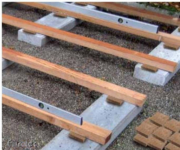
The cork pad spacers are laid between the deck substructure and the foundation/subsurface (self-adhesive on one side) and thus form a gap that aids constructive timber protection. The cork pad spacers are available in three sizes. These are 3 mm, 6 mm and 10 mm thickness/height (see Fig.). In addition to the advantages already mentioned, useful side effects of using the spacer include the option to adjust the height of the substructure and that the loads are distributed evenly.
