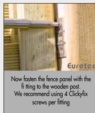
Now fasten the fence panel with the fitting to the wooden post. We recommend using 4 Clickyfix screws per fitting
