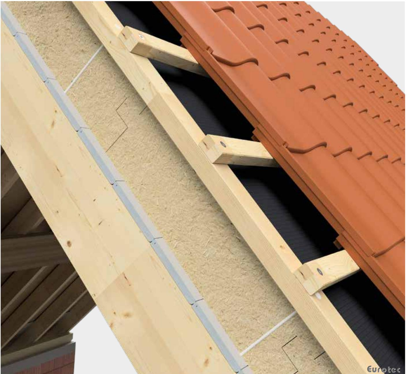
Only suitable for insulating materials  $\geq 50$  kPa (pressure-resistant)
